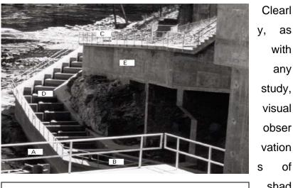
Figure 32. Brunswick fishway; (A) location of river observations, (B) lower fishway, (C) corner pool, (D) pool 14, (E) upper fishway - pool 31.
