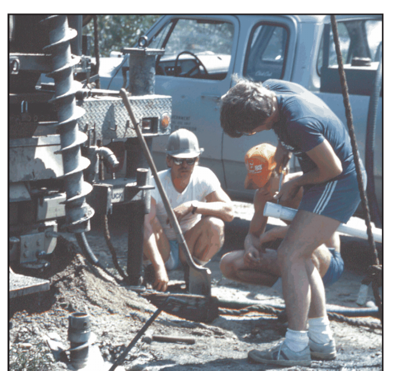
Installing a monitoring well, Washington County, Maine.
