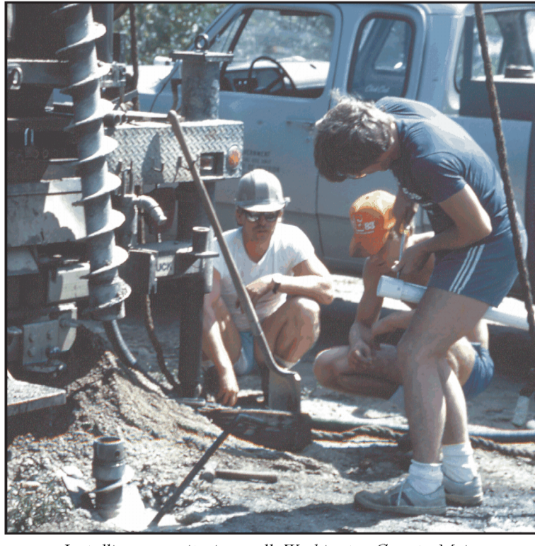
Installing a monitoring well, Washington County, Maine.
