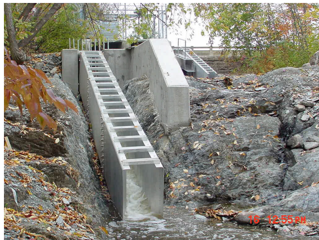
Figure 5. Alaskan Steppass Fishways at Plymouth Pond Outlet Dam, October 2002
