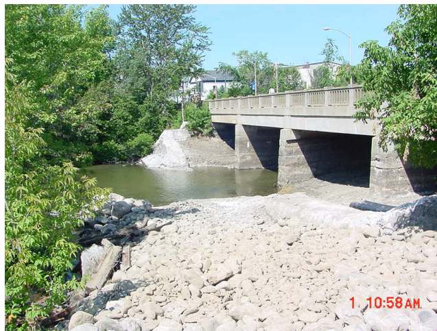
Figure 6. Site of the Former Guilford Dam, August 2002
