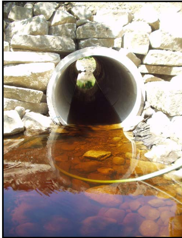
Photo 2. External Structure Ponding Water into Smooth-bore Slipline to provide adequate depth and low water velocities. Route 27 over unnamed tributary to Carrabassett River, Carrabassett Valley, Maine. Target Species: brook trout.
