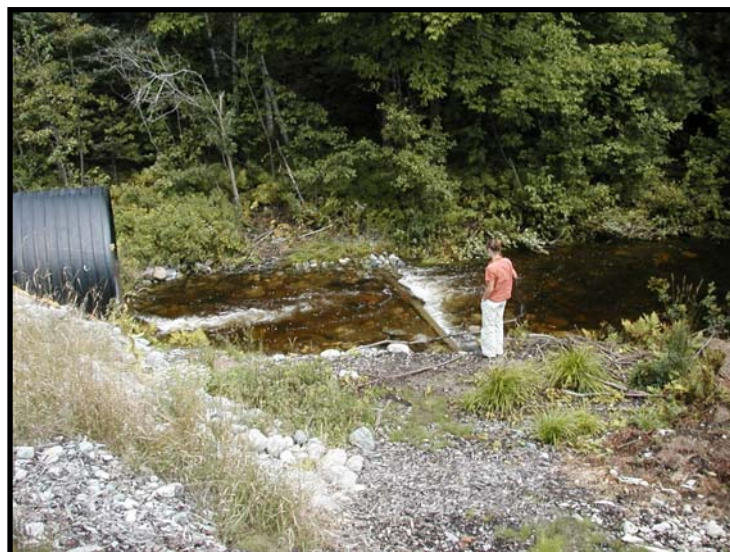
Photo 2. External Structure Ponding Water into Smooth-bore Slipline to provide adequate depth and low water velocities. Route 27 over unnamed tributary to Carrabassett River, Carrabassett Valley, Maine. Target Species: brook trout.
