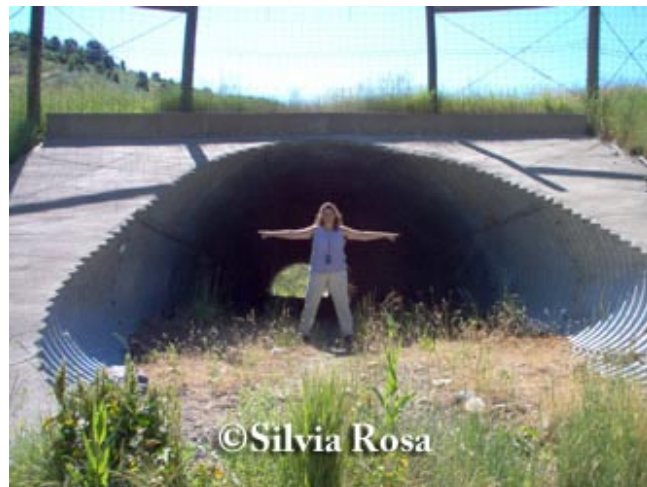
Figure 11. Medium-sized mammal passage under US Route 89/91. Utah .
