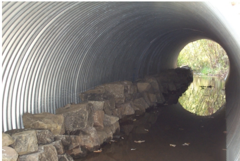
Figure 12. Medium-sized mammal passage under Territorial Highway. Loraine, Oregon. Photo by John Levenhagen
