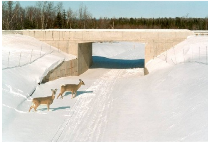
Figure 9. Small bridge span for large wildlife passage. New Brunswick. Photo courtesy of NBDOT
