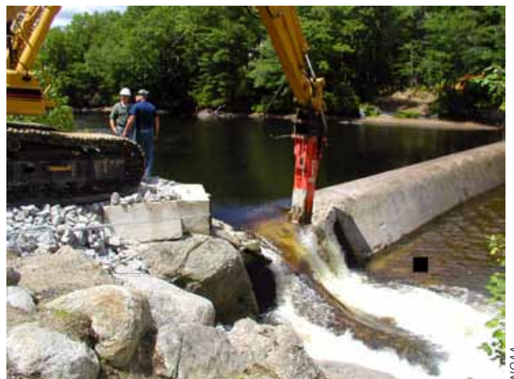
Removal of aging, unneeded dams provides many benefits for fish and wildlife, and for overall ecosystem health.
