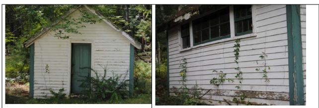
**Condition:** Fair to poor. Sills appear compromised. Roof in poor condition.
