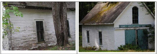
**Condition:** Fair to poor. Sills appear compromised. Roof in poor condition.
