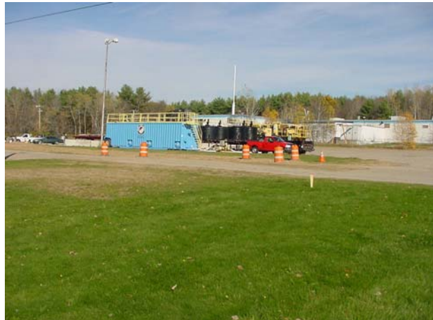
Figure 44. The processing plant set up in the Maine Electronics parking lot.
