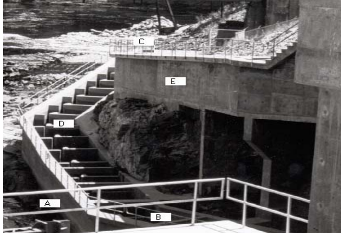
Figure 32. Brunswick fishway; (A) location of river observations, (B) lower fishway, (C) corner pool, (D) pool 14, (E) upper fishway - pool 31.
