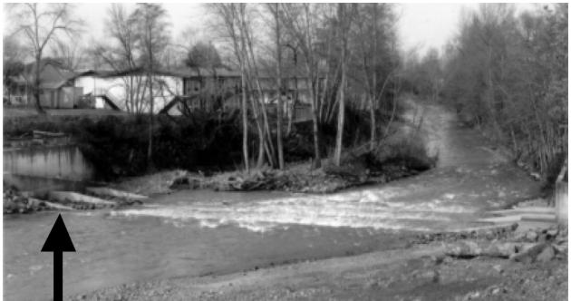
The concrete wall on the left bank is what remains of the original diversion dam.
