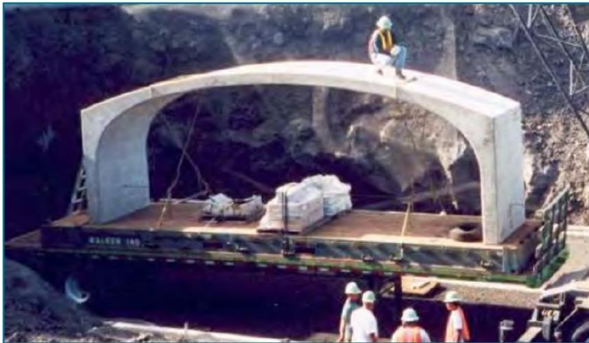
FIGURE B.9 - A three-sided rigid frame section. Image source: Precast Solutions.
