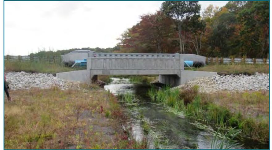
FIGURE B.6- A three-sided concrete rigid frame structure, installed on pre-cast footings. Clear span of 24 feet. Structure includes a pre-cast modular design with six-foot-long sections. Due to cover limitations within the road prism, an insulated water line was attached to side of headwall. Coonamessett River, Falmouth, MA. Image source: Inter-Fluve.
