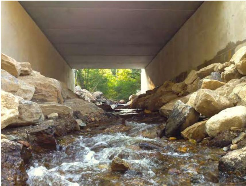
FIGURE 5.3 - This MaineDOT crossing was designed to adequately accommodate storm flows, protect footings from scour, facilitate low-flow water depths sufficient for fish passage, and allow for semi-aquatic wildlife movements. Photo by Slade Moore.
