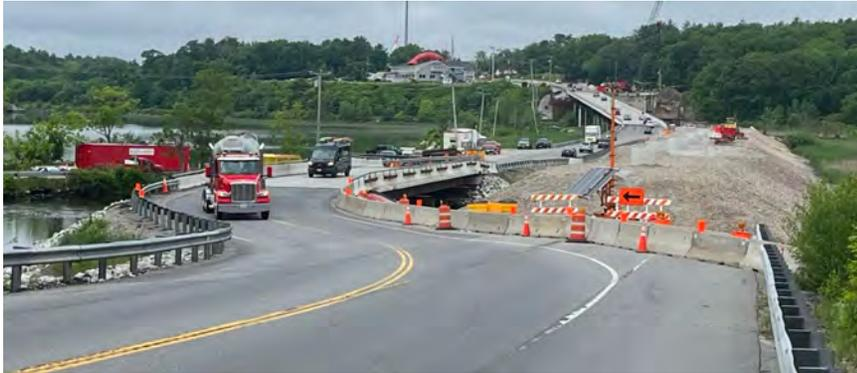
FIGURE 8.1 - When tidal crossings are replaced in primary traffic corridors, temporary traffic bypasses may be required. This temporary bypass along Route 1 in Woolwich, Maine, was used during bridge replacement and construction to restore tidal flow to Back River Creek Marsh. Photo by Michael Burke.
