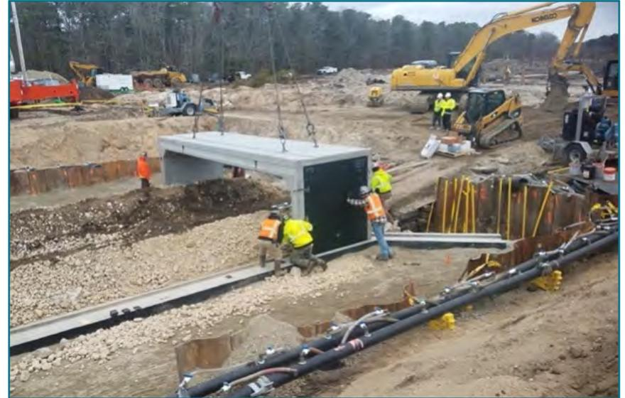
FIGURE B.10 - A three-sided rigid frame section being installed on pre-cast footings. Coonamessett River, Falmouth, MA. Image source: Betsy Gladfelter.
