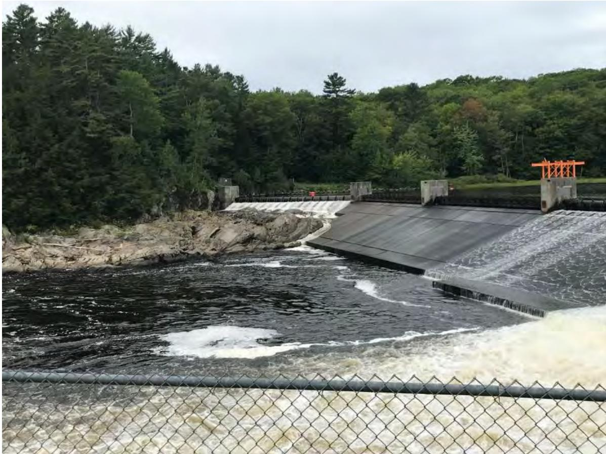
**Figure 5.0-2: Bascule Gate No. 5 in Fully Lowered Position (9:37 am)**
