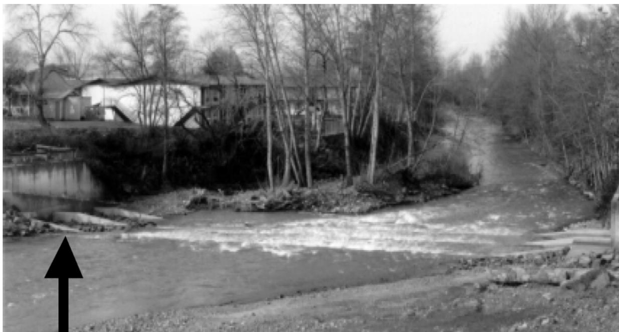
The concrete wall on the left bank is what remains of the original diversion dam.
