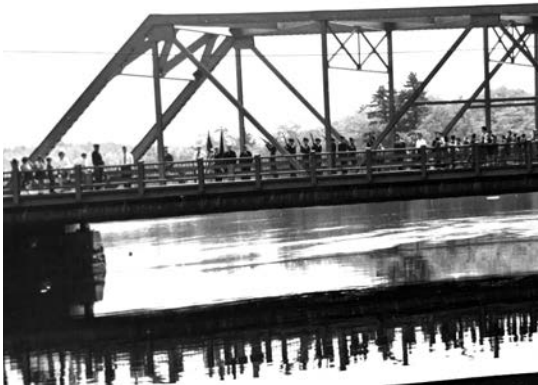
The Green Bridge:
