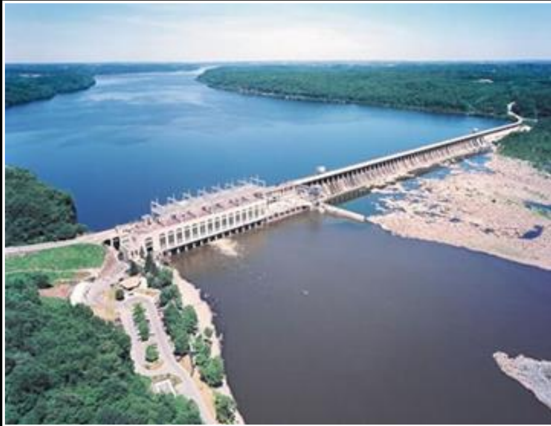
Conowingo Dam, Susquehanna River
